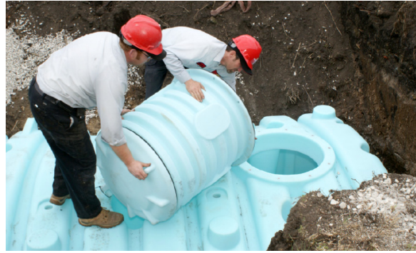
Workers install green infrastructure at a former brownfield site
