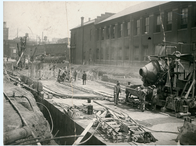
Far left: A view from Pogue's Run in Brookside Park. Left: Construction crews work to build the Pogue's Run box culvert in 1914. Above: Pogue's Run entering the double box culvert at New York Street
